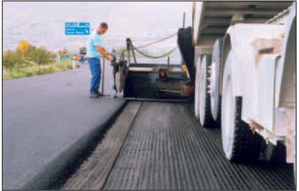
Installation of HaTelit® southern Spain 1999
